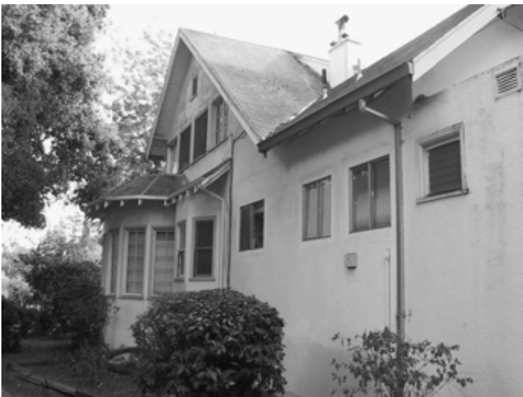
Figure 24: Right side view, 80 Finger Avenue, showing 1935 addition at rear
