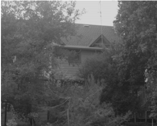
Figure 15: Dormers on eastern wall; windows have been moved
