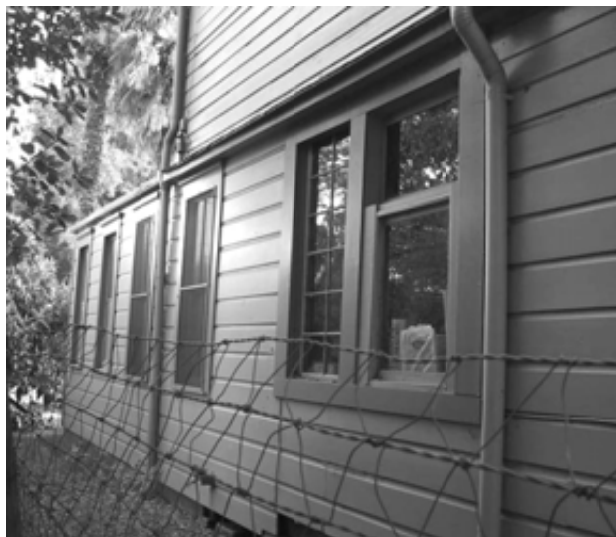
Figure 14: Ground floor, addition on eastern side
