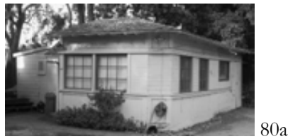
80a Finger Ave., Garage/Residence (after 1930)
