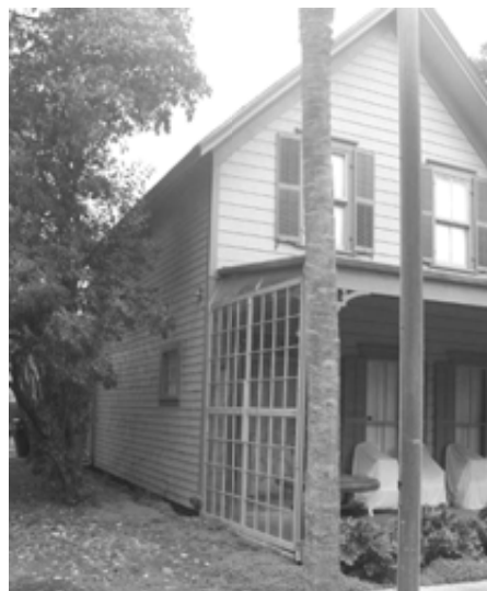
Figure 11: Shingles on western side where original house section was removed (side wall to left in photograph)
